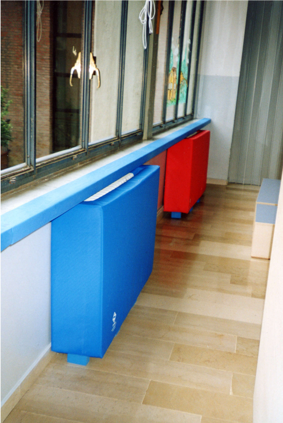
RADIATOR STUFFED PROTECTION
